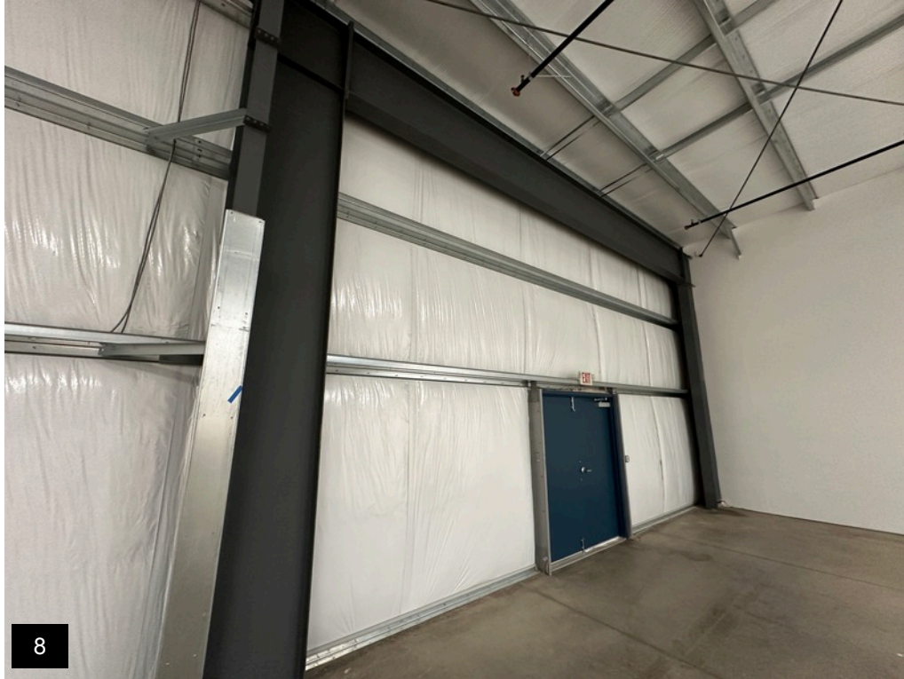
The typical longitudinal steel moment frame.
