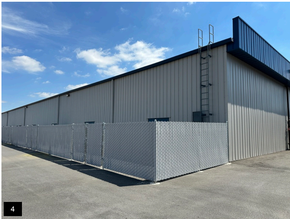
The typical steel light framed rear elevation.
