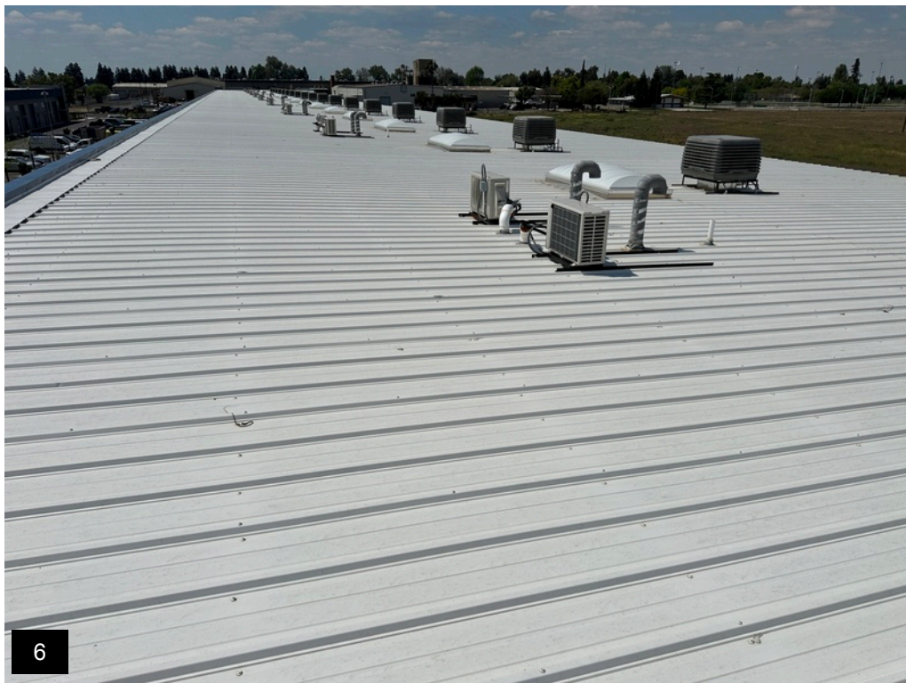
The typical corrugated metal roofing.
