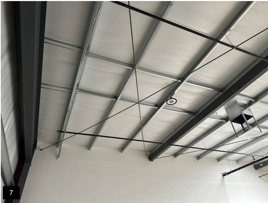
The typical roof tension-only cable diaphragm bracing.
